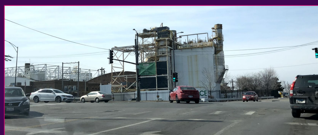
This picture depicts a petroleum refining plant. The banner proudly reads that the Grace Plant is celebrating its 75th anniversary in this community. Their website highlights their "community partnerships," one of which is with UIC.
